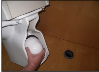
2 – Install the discharge pipe
