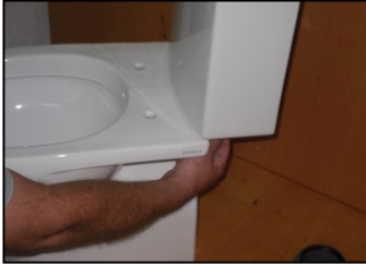
1 – Install the ceramic reservoir
