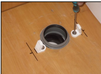
7 – Install floor mounting kit
