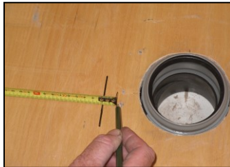
5 – Add basin wall thickness 12mm
