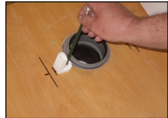
6 – Mark the center of the fixing holes
